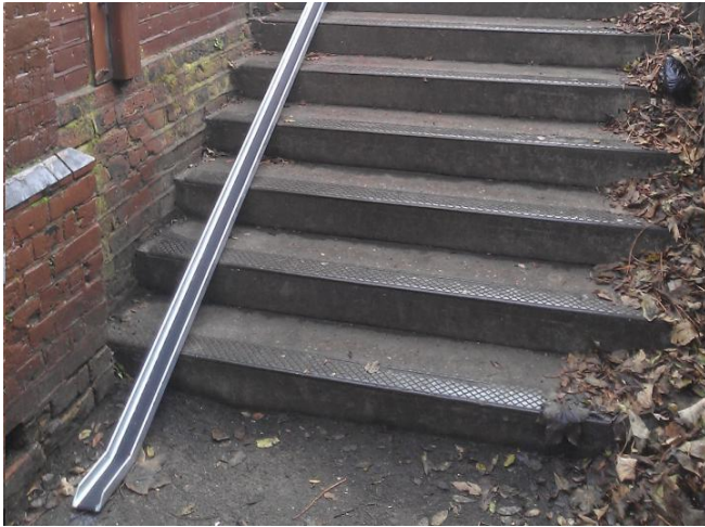
Example of cycle ramp installed in 2010 at Queensmead Road Bridge.
